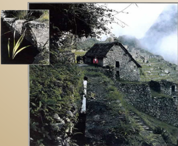
Photograph 2. The Inca supply canal flowed gently into Machu Picchu at an engineered grade on a carefully built terraced right-of-way.
