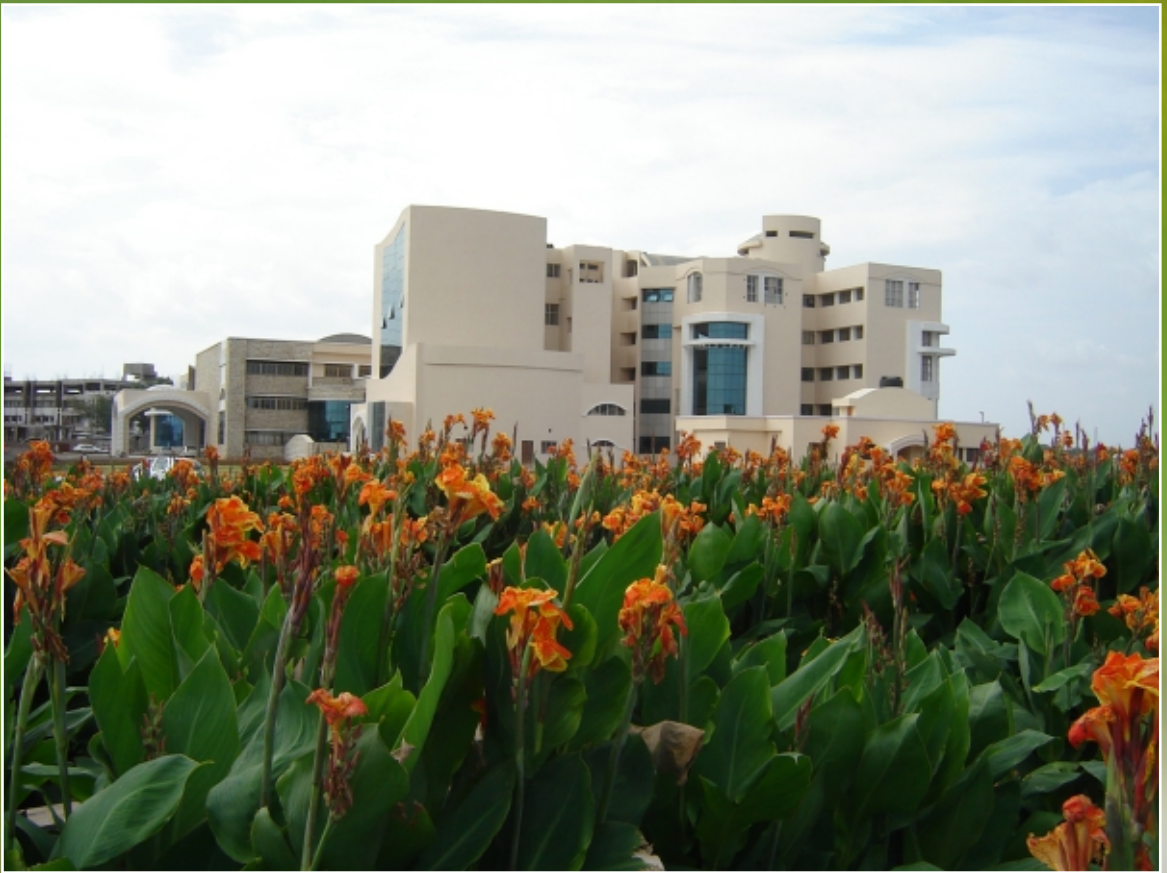
SIBF system at Bharati Hospital and Medical College, Sangli
