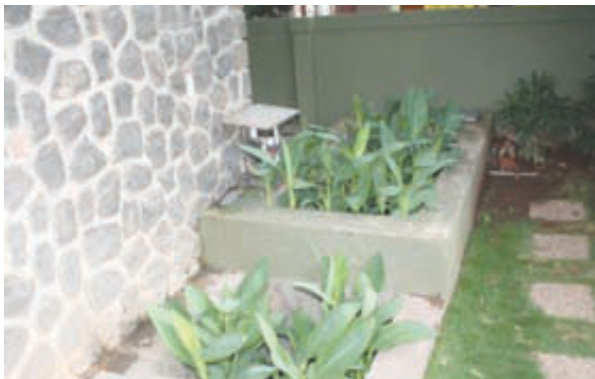
▶ SIBF system employed for water recycling.
