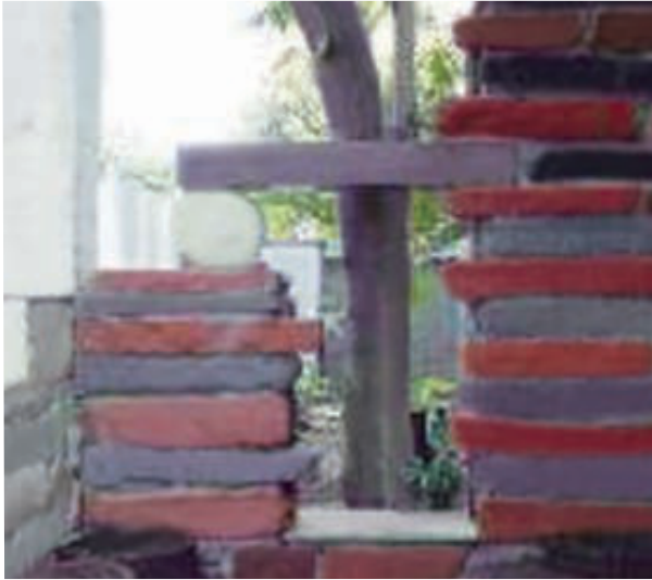
► The separation wall topped by a flat marble stone resting on a concrete sphere.
