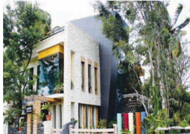
▶ The compound wall has been constructed by cohesively bringing together various waste materials collected from other construction sites.
