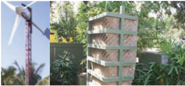
▶ Windmills on the roof and wind-catcher (part of the Earth tunnel) in the compound to aid air-conditioning.
