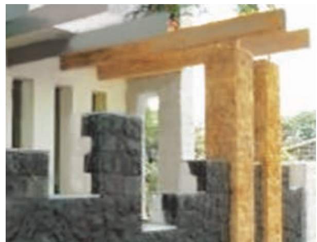
▶ At the Entrance: The focal point of the elevation is a pair of yellow 'Rabkavi' stone pillars.
