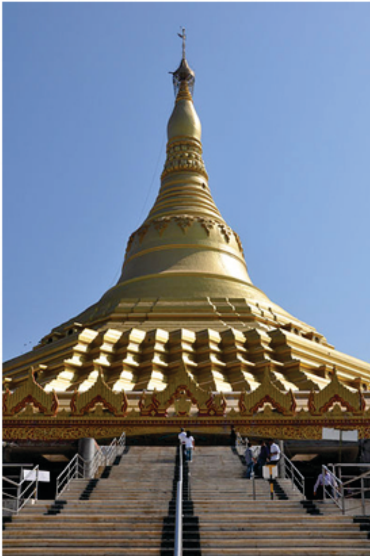
View of the main marble stairway
