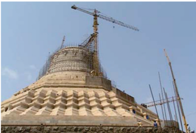
Catenary dome in progress
