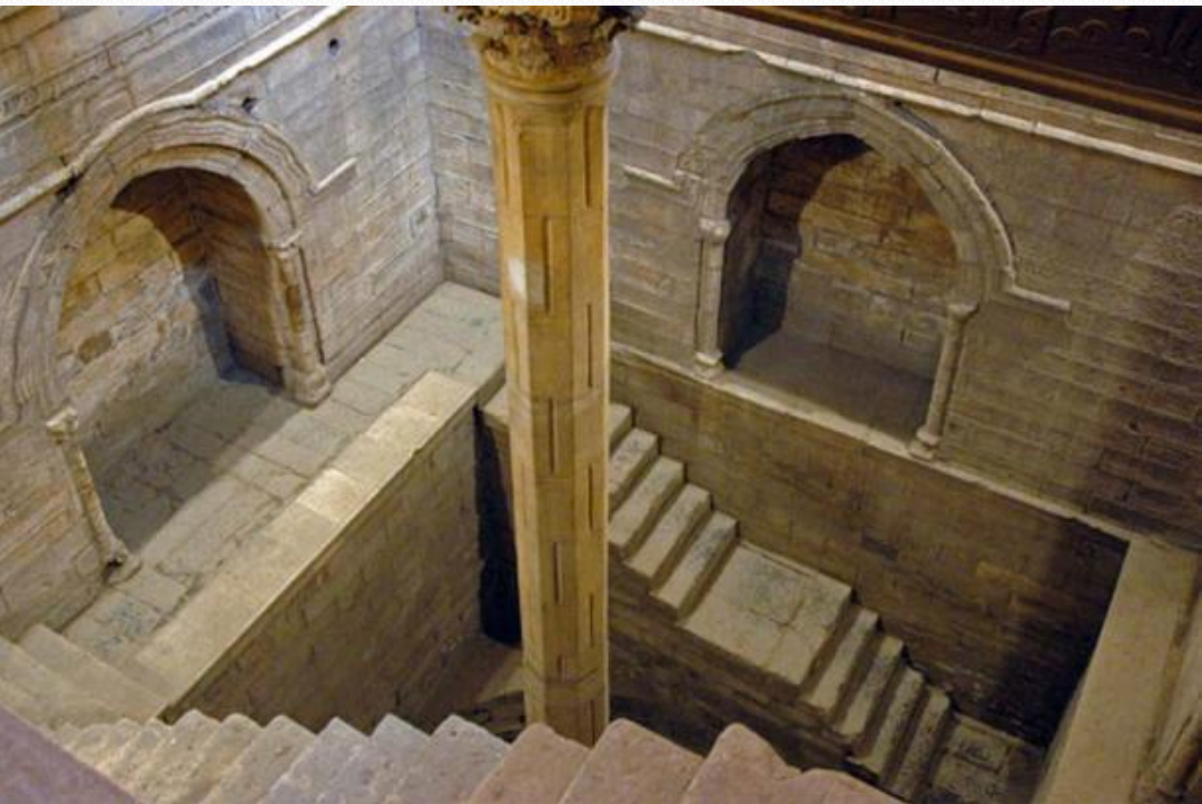
Measuring shaft of the Nilometer on Rhoda Island, Cairo. Nilometers measured how high or low the flood would be. ( CC BY-SA 3.0 )
